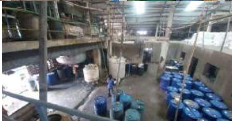
Openly stored drums filled with various materials near ETP area and in plant area
