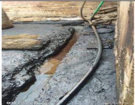
Drain to carry waste water generated from plant to ETP area
