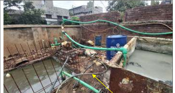
Material was transferred by AOD Pump connected with Separator Vessel and a flexible pipeline open at ETP
