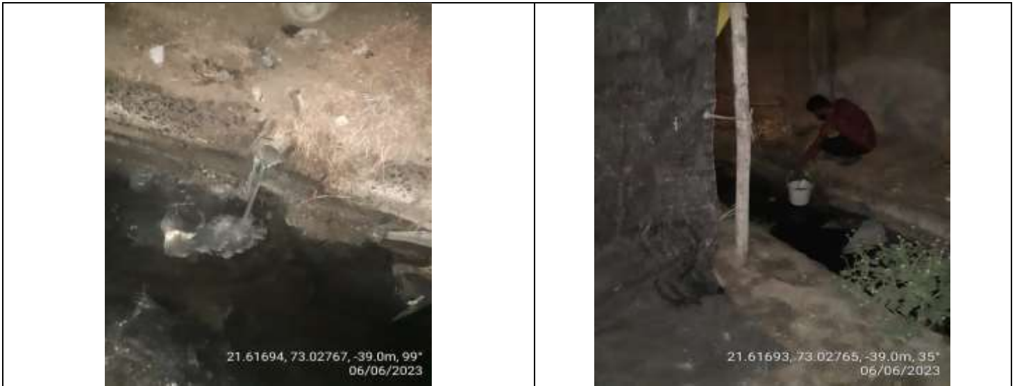
Alkaline and highly odor containing w/w discharge is going on from the outlet of discharge pipe line provided in the Bathroom of M/s. Shchem Corporation.
