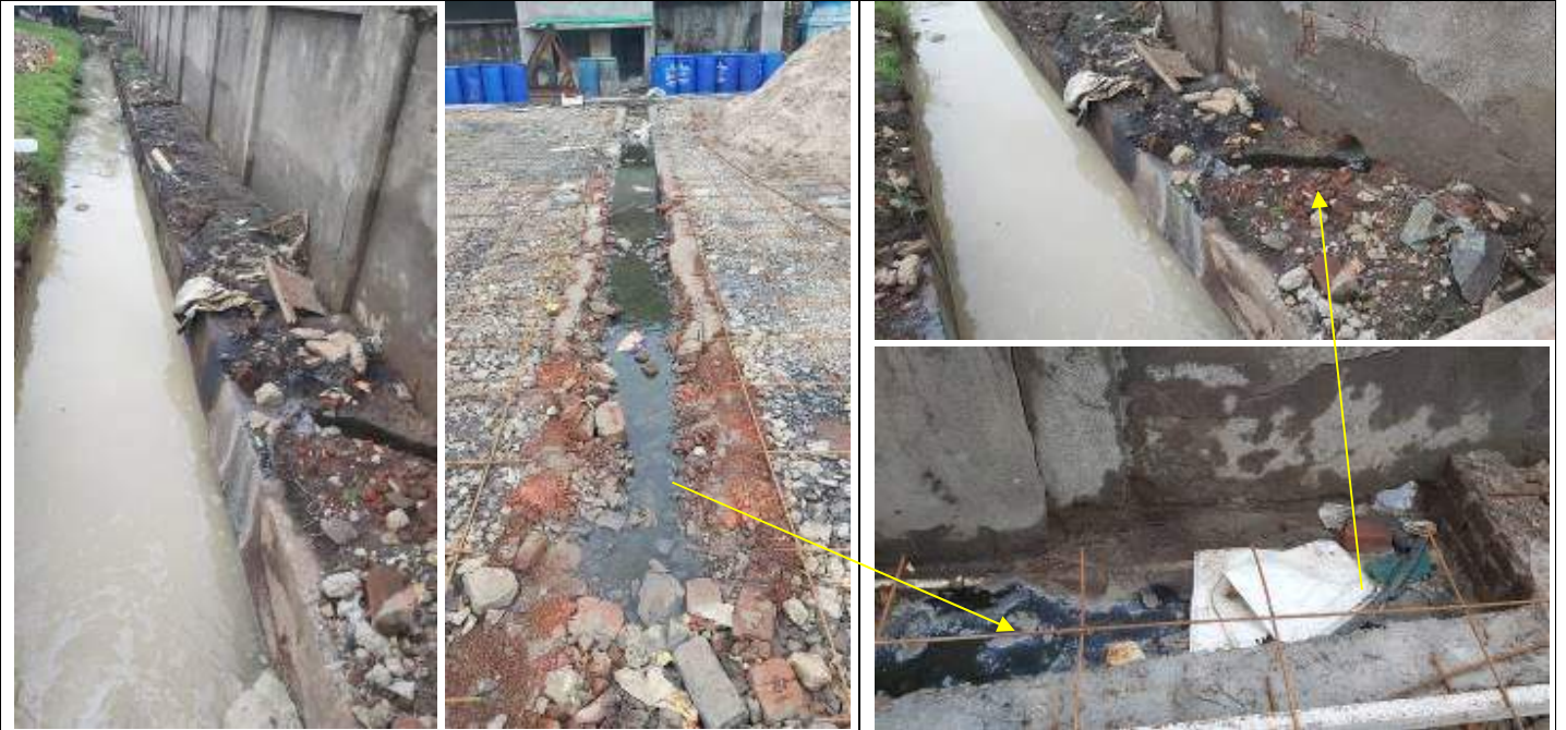
Contaminated alkaline wastewater going outside through boundary hole near material gate
