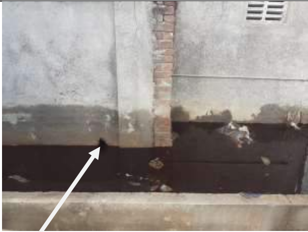
One Hole provided in boundary wall for disposal of w/w and Alkaline w/w ponding is observed outside of the unit premises.
