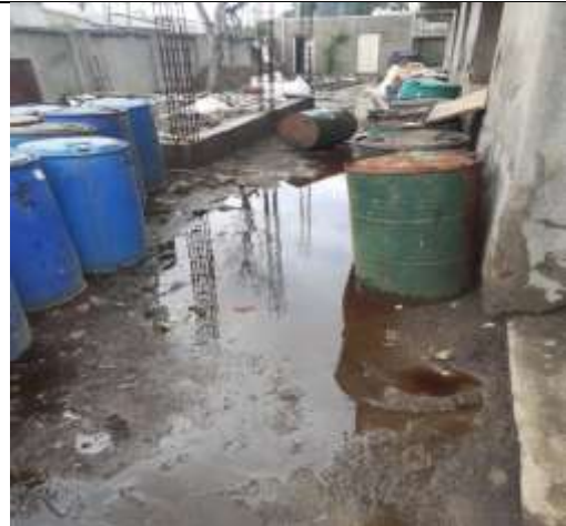
Alkaline w/w ponding is observed within the unit premises.
