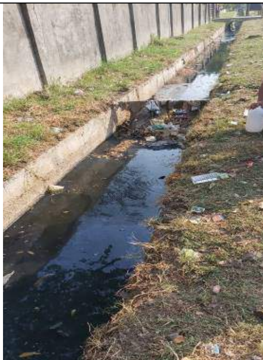
GIDC storm water drain outside the premises mix with other streams mostly domestic waste water pH found alkaline
