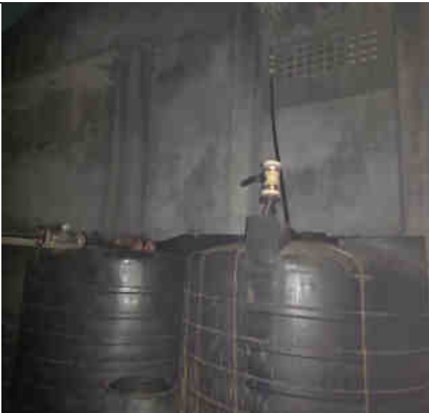
Flexible pipeline is coming from reaction vessel to final treated w/w holding cum CTEP disposal tank and Flexible pipe line with pump is provided in the bottom of both final treated w/w holding cum CTEP disposal tank.
