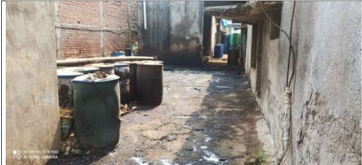
Poor housekeeping near ETP Area
