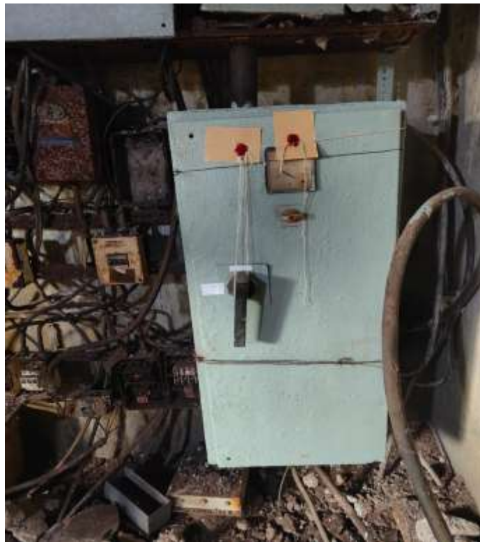
Main electric panel board by switching off main electric switch is sealed
