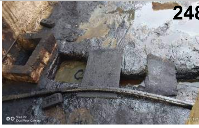
Drain to carry waste water generated from plant to ETP area
