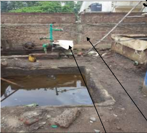
Collection tank of ETP with Electric motor pump with flexible pipe line up to the open land at backside of the unit as disposal facility for untreated w/w disposal
