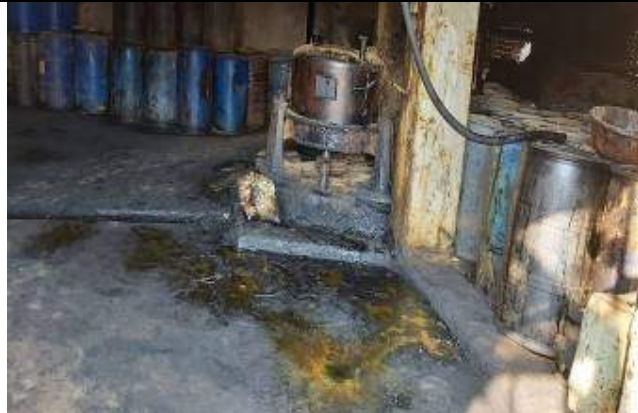
Drain to carry waste water generated from plant to ETP area
